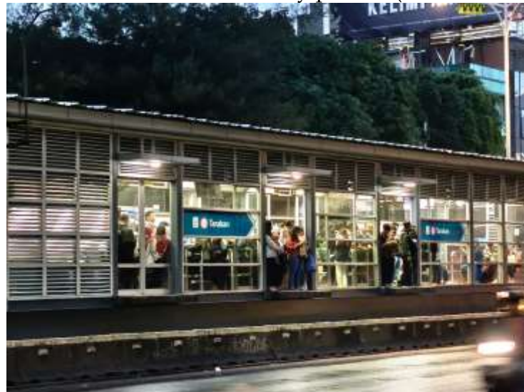
Figure 5. Bus Shelter Seen from Outside
